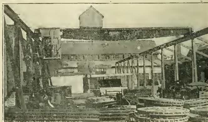
STOREHOUSE YARD CRANE.
